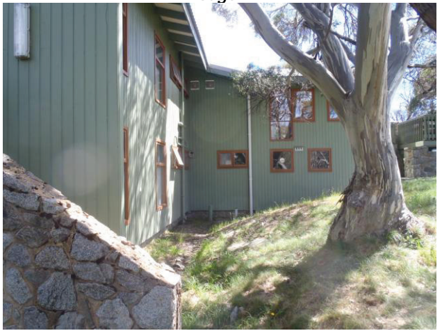
Figure 7: Photo of the south-eastern corner of the lodge
